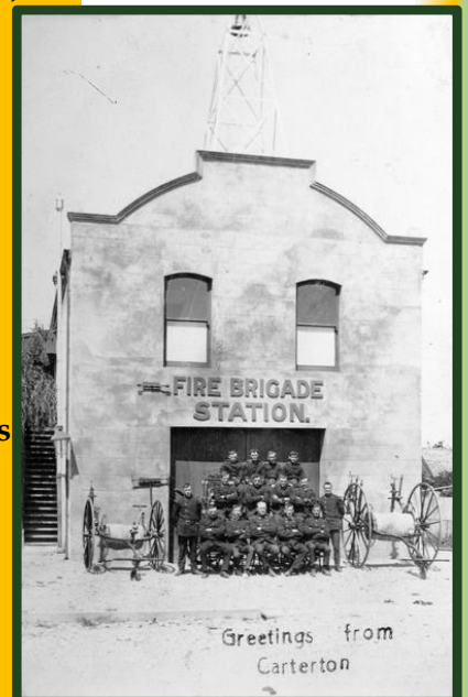
Carterton Fire Brigade Station 62 Constructed in 1906
